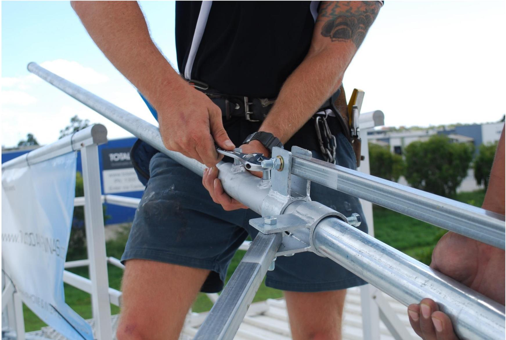
18. Determine position of second strut baseplate (approx. 2m from mast base at 90° to each other)..
