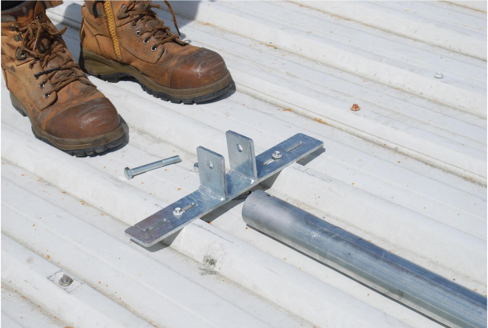
6. Slide collar of adjustable stay bar onto the base section of mast.
