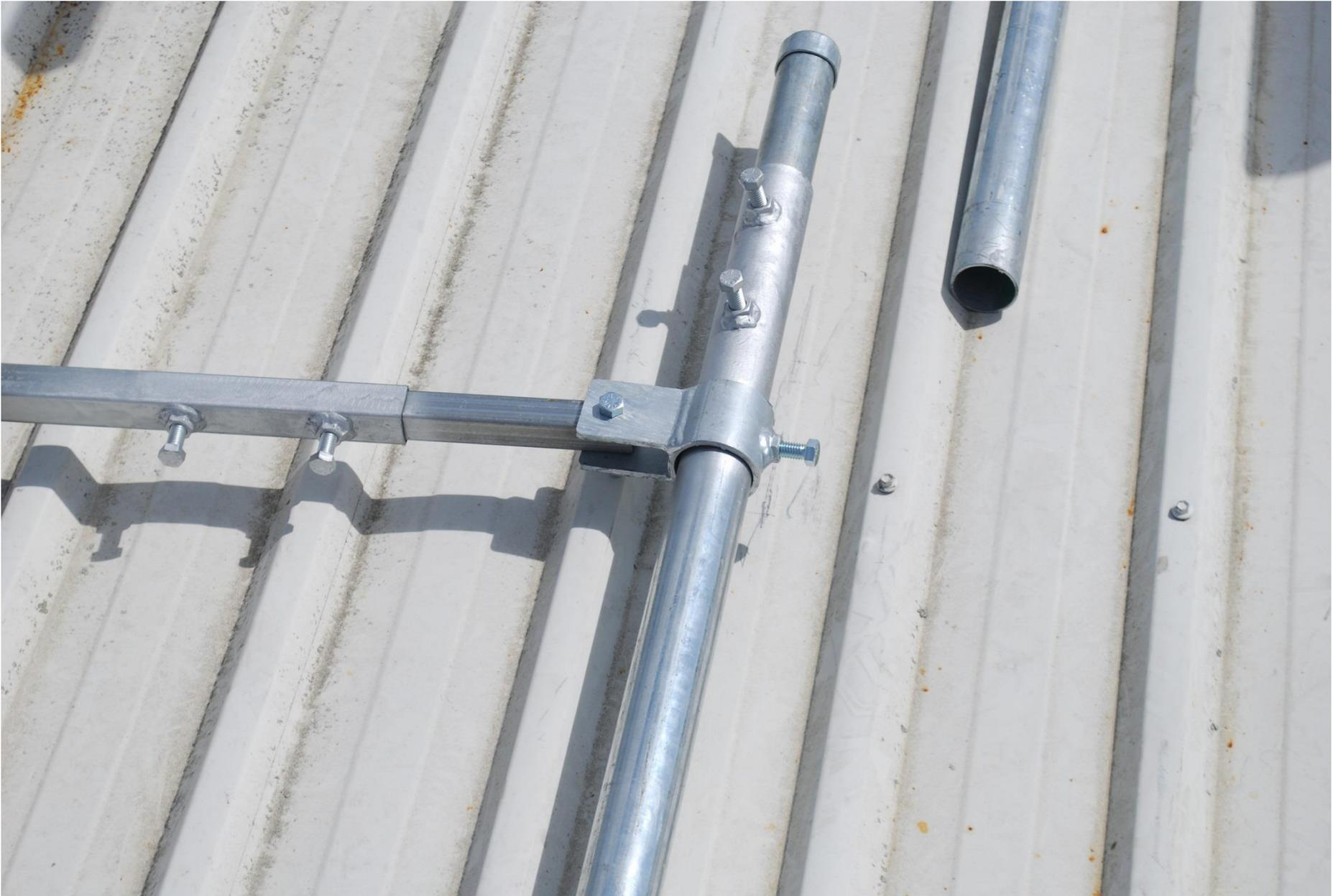
8. Tighten collars onto mast to prevent slipping but allowing for manual re-orientation.
