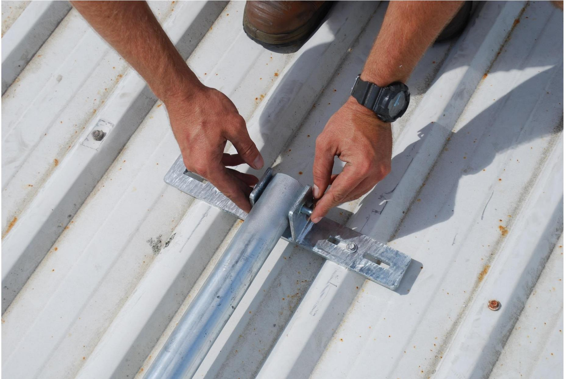
12. Determine position of first strut baseplate (approx. 2m from mast base at 90° to each other).
