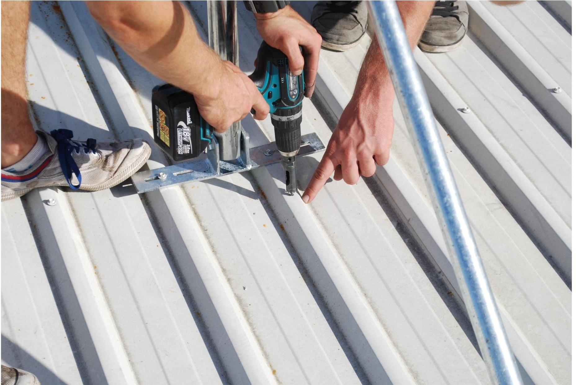
12. Cut hole in roof to suit diameter of conduit.
