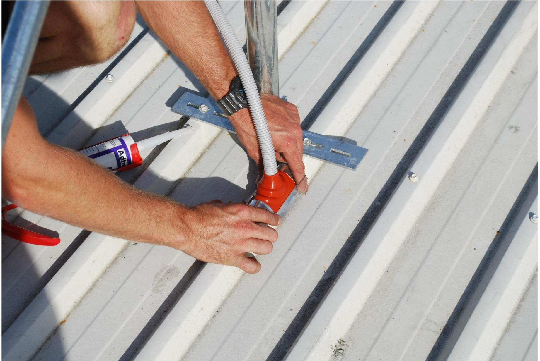
19. Fix flashing to roof with screws.
