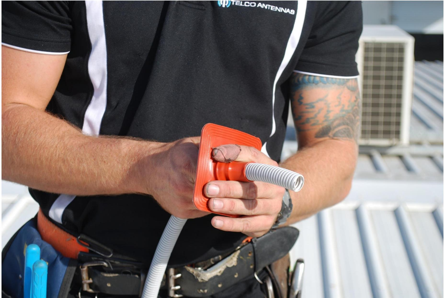
15. Feed conduit through roof penetration.
