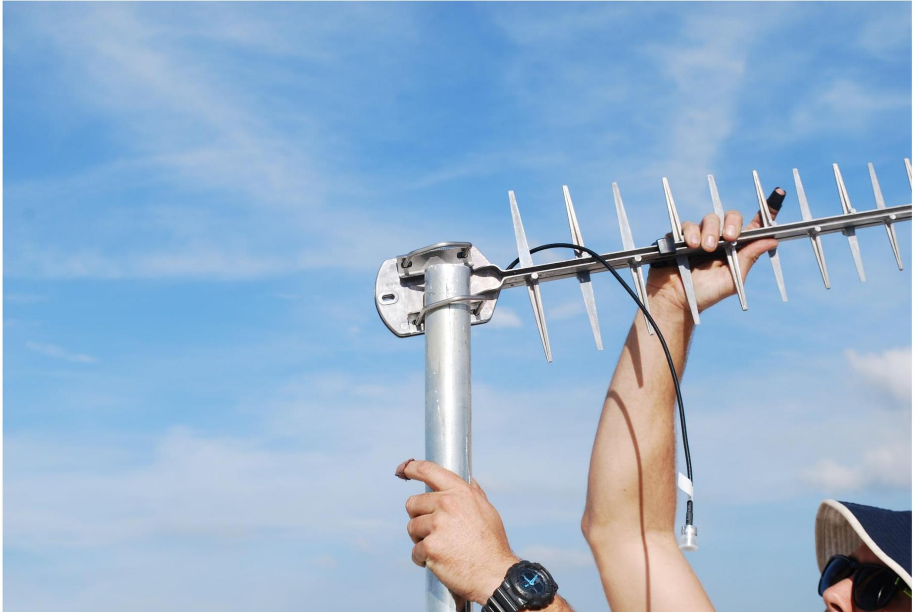
6. Tighten nuts allowing enough give to rotate/adjust.
