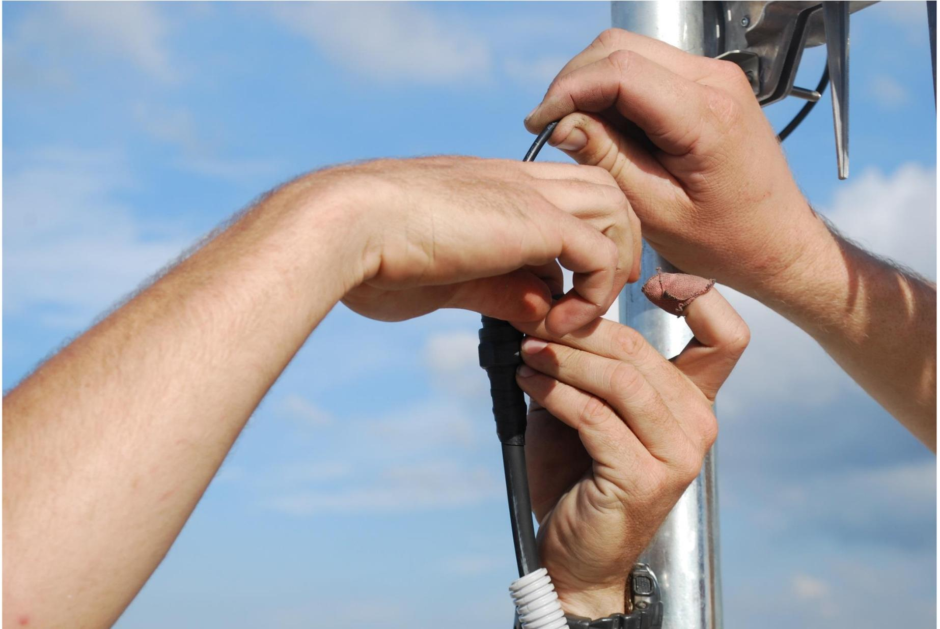
30. Slide connection to top of conduit and cover with tape.
