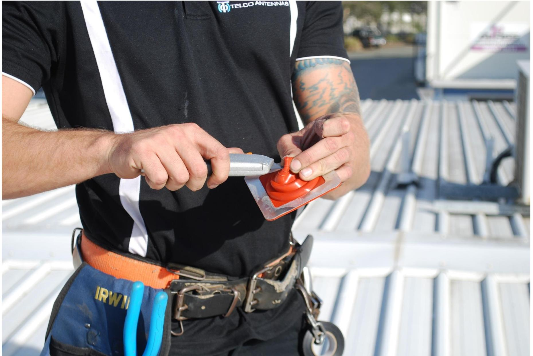
14. Feed conduit through flashing.
