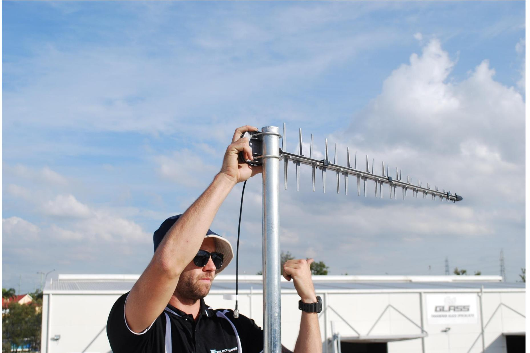
8. Align antenna to tower and tighten bracket.
