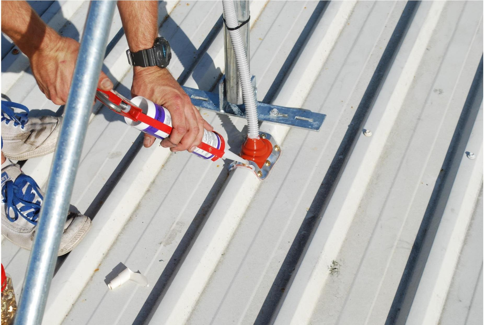
36. Ensure all gaps are covered with silicone (including the screw penetrations of mast).
