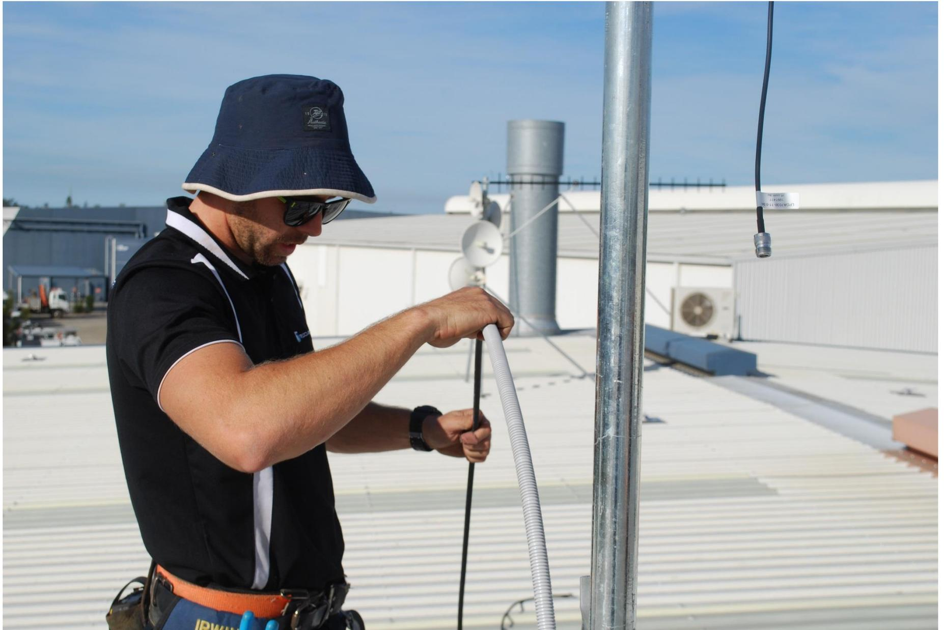
23. Attach conduit to mast with cable ties.
