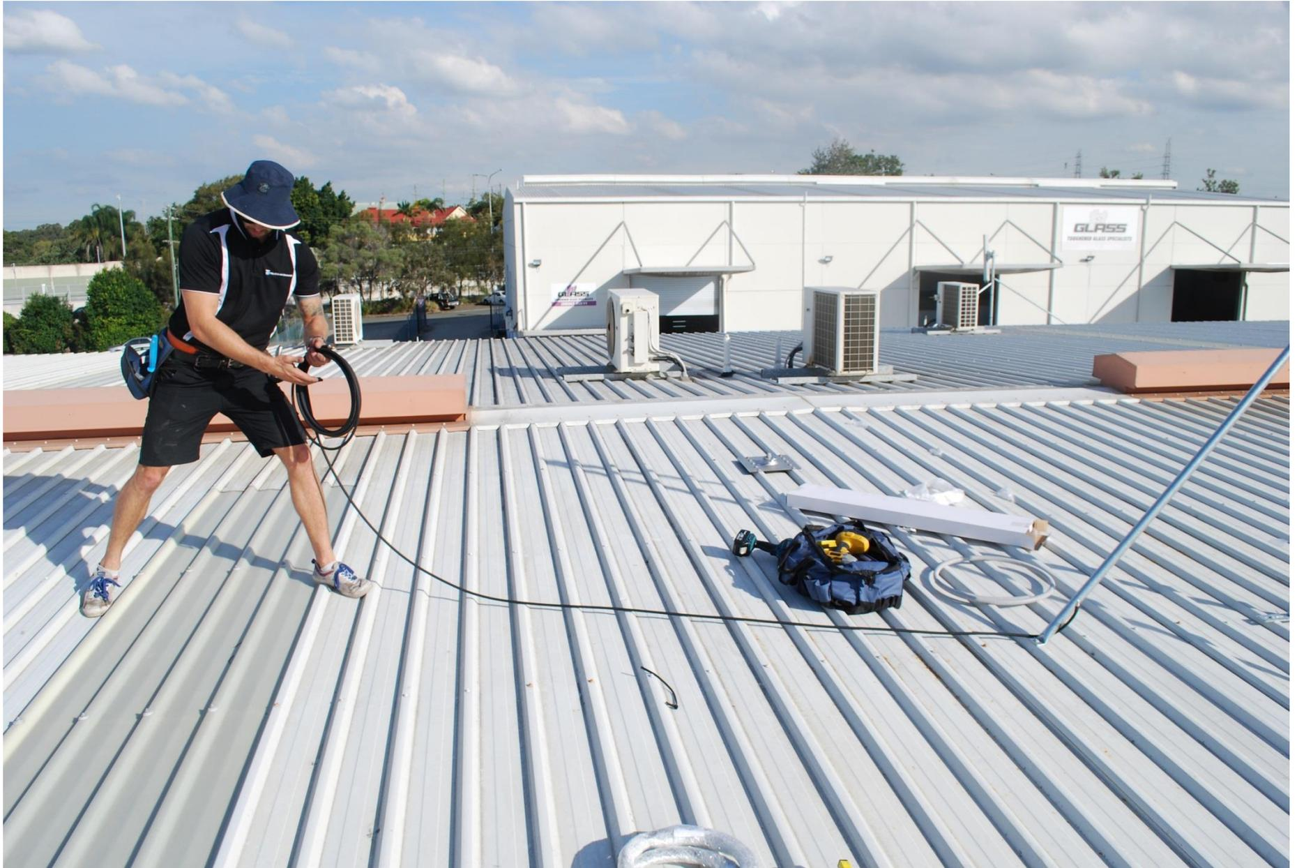
11. Determine location of roof penetration (**on a crest not in a trough**).
