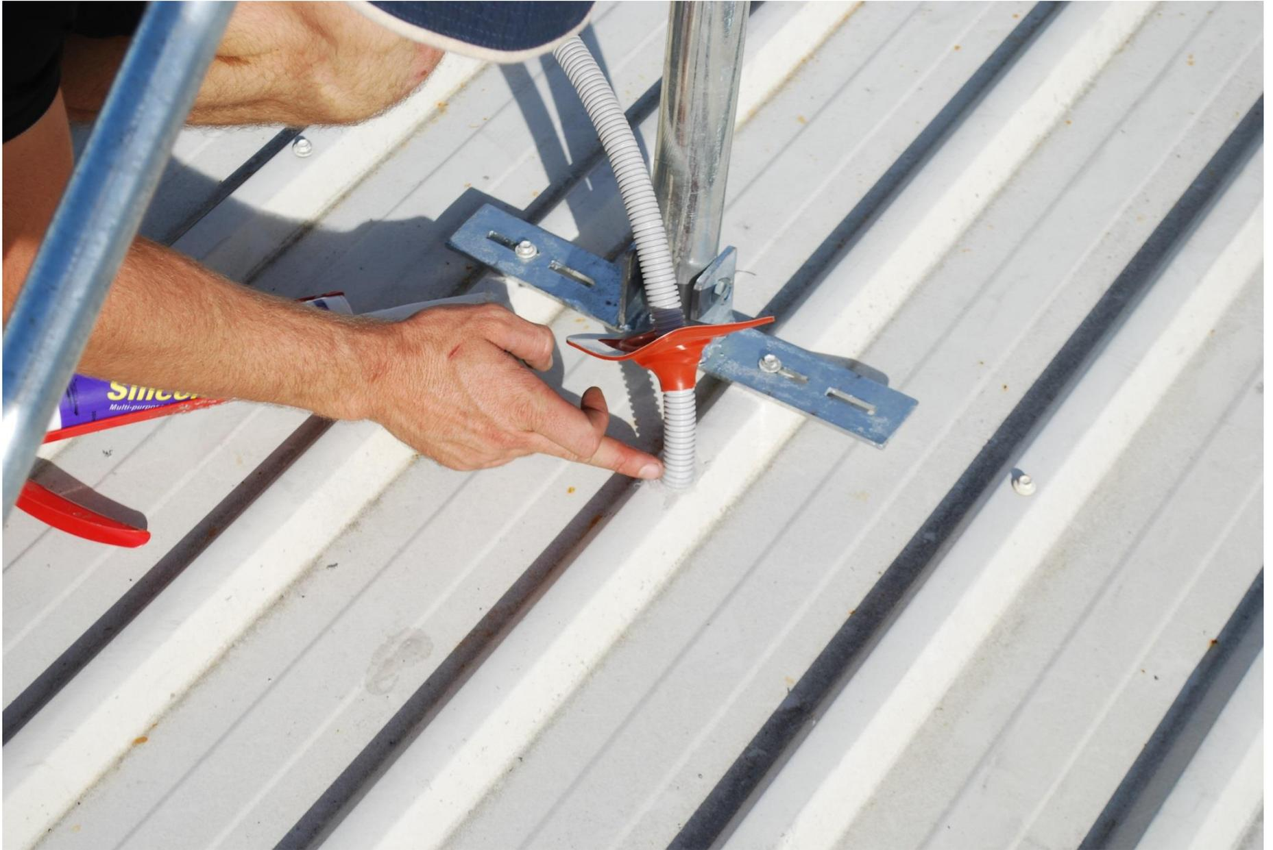
18. Mould flashing to suit contour of roof.
