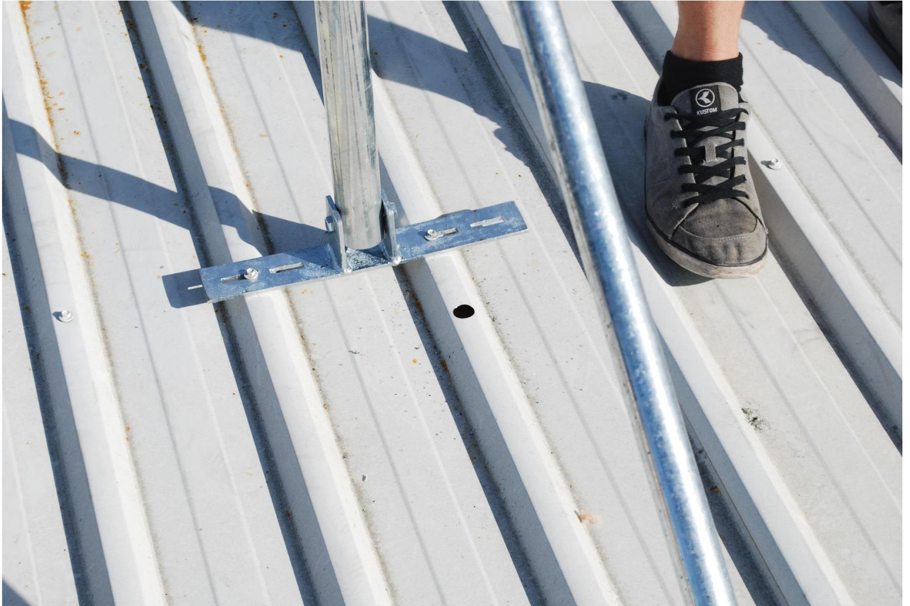
13. Cut roof flashing to suit diameter of conduit.
